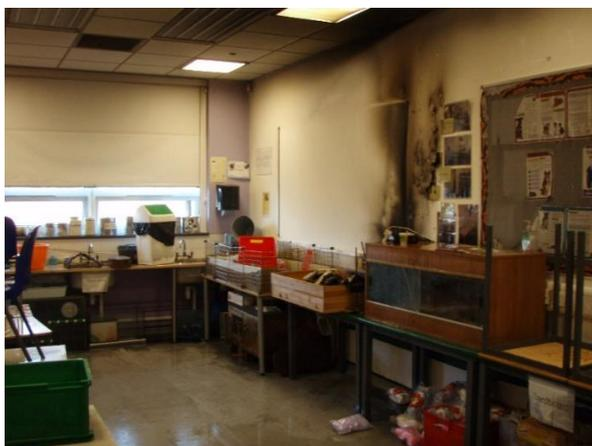
An electric heat lamp in the animal care classroom of a Newcastle school malfunctioned causing a fire with over 200 people on-site. One sprinkler head activated which confined the damage to the room of origin and extinguished the fire. A number of small animals were in the room involved and all survived whilst no other areas of the school were affected. Damage was limited to a wooden bench and minor smoke damage amounting to less than 1% of the whole building. Damage was repaired quickly.
